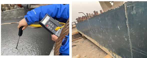
图10 UHPC浇筑温度测试 Fig. 10 UHPC pouring temperature test Fig. 11 UHPC formwork removal appearance
