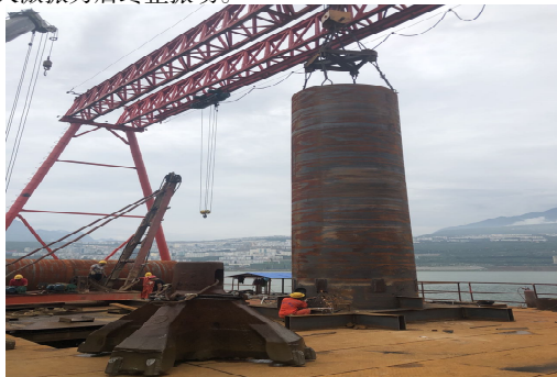
图 7 钢护筒对接 Figure 7 Docking steel casing
