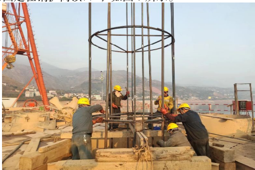
图 8 钢筋吊笼 Figure 8 Hoisting steel reinforcement cage
